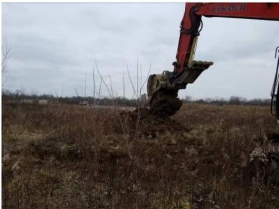
Photo #5: View of staging of test pitted soils for sampling (1/6/2021).
