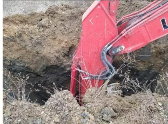
Photo #2: Further example view of test pitting of stockpiled soils (1/6/2021).
