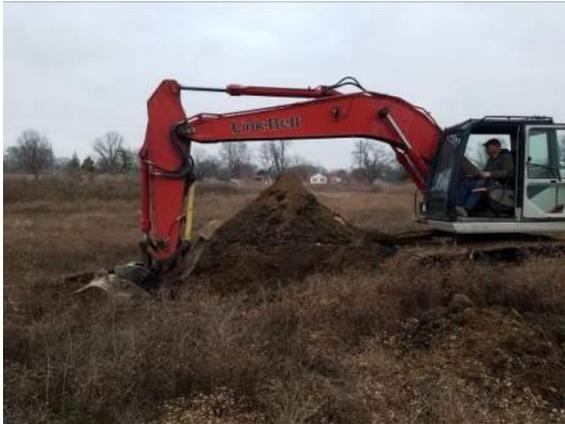
Photo #1: Example view of test pitting of stockpiled soils (1/6/2021).
