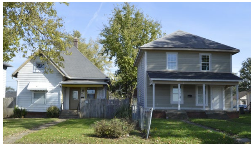
Existing residential homes near the Sherman Park site.
